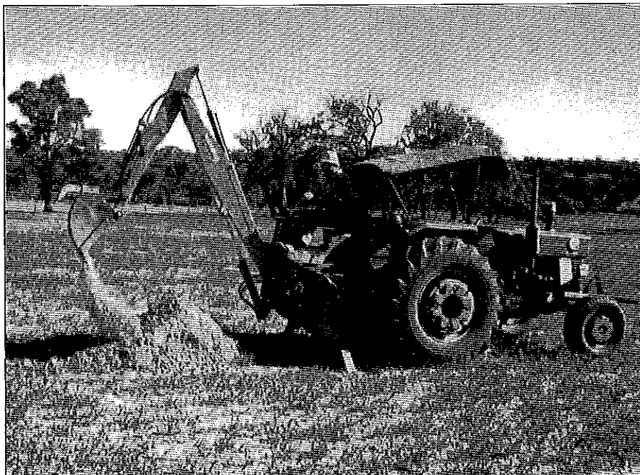
Figure 3.13 How to use a backhoe to dig a soil pit.
